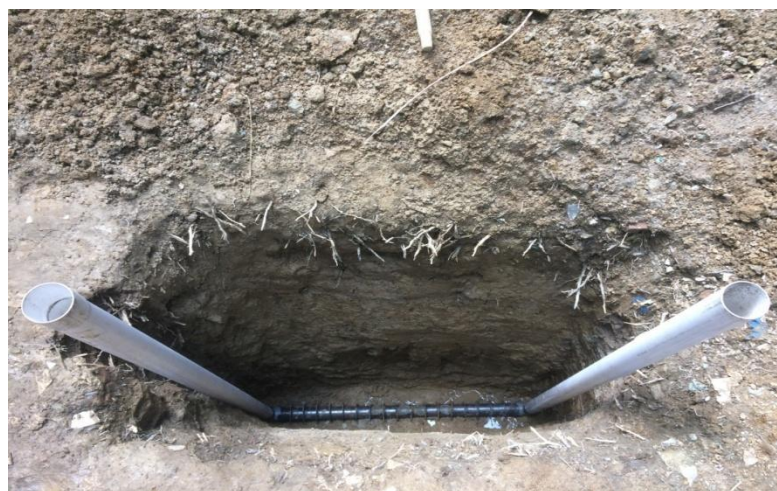
Figure 2. An EAHE in the ground
