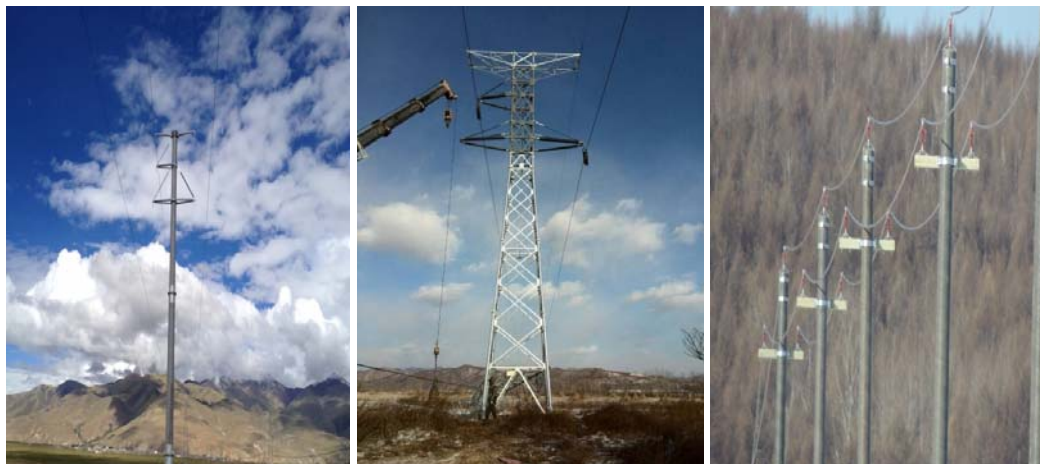
Figure 1. NARI 110kV FRP composite pole (left) ,220kV truss tower(middle) and 10kV crossarms and poles (right) manufactured with PUP resin.
