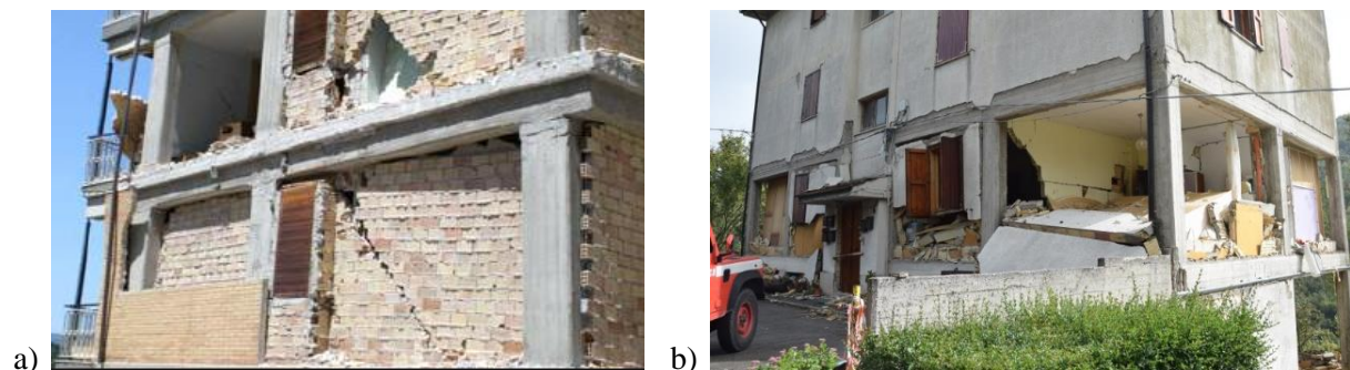
Figure 2. Examples of infill failure: cracking and corner crushing (a), out-of-plane movement (b).
