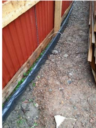
Figure 4. Applied fence of the construction site to prevent migration of water [07.11.2016]
