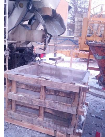
Figure 5. Recovering the concrete mix by means of a filter basket during the washing trough truck mixer [19.01.2017]
