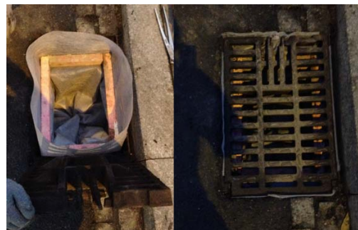
Figure 7. An example of securing manholes using a geotextile basket [25.09.2016]
