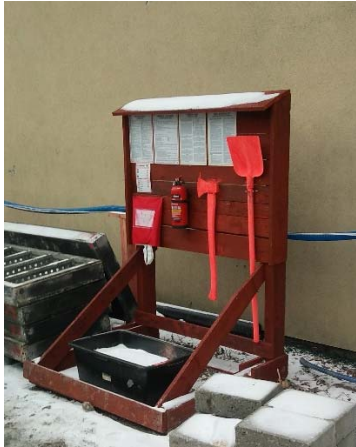
Figure 3. Prepared fire station [19.01.2017]
