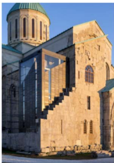
Figure 8. The Fragment of the Bagrati Cathedral, the western facade with the built-on elevator shaft, [3]
