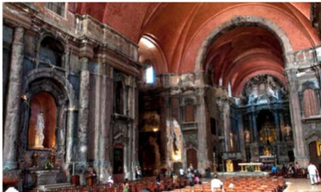
Figure 7. The Church Interior after renovation, the current state of the Church (photograph by B. Pierścioneck)
