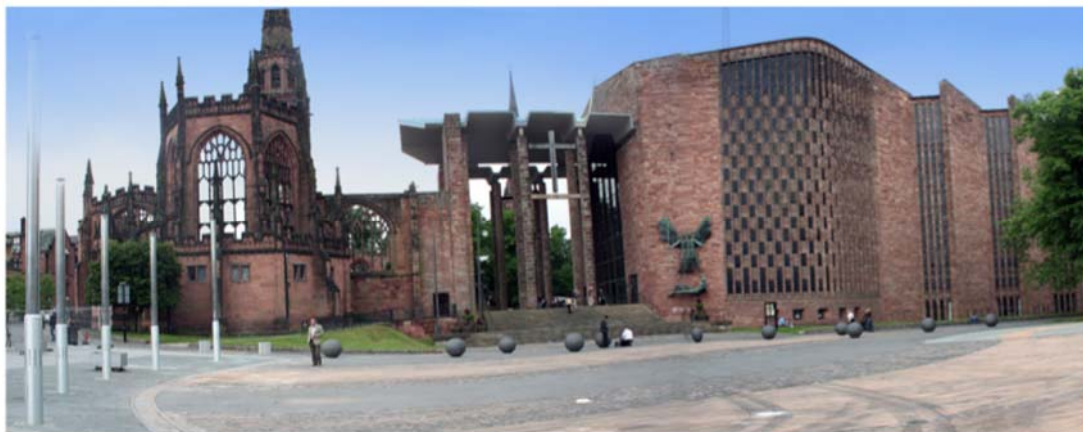
Figure 3. St Michael's Cathedral in Coventry. The Medieval fragment is on the left-hand side, and the contemporary fragment - on the right-hand side
