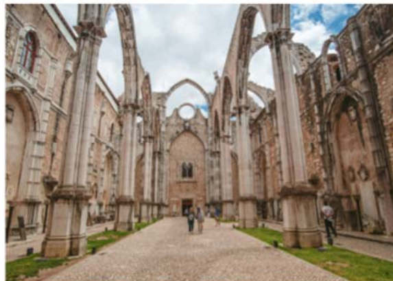
Figure 5. The Interior of the Church preserved in the form of sustainable ruins, the current state of the ruins (photograph by B. Pierścioneck)
