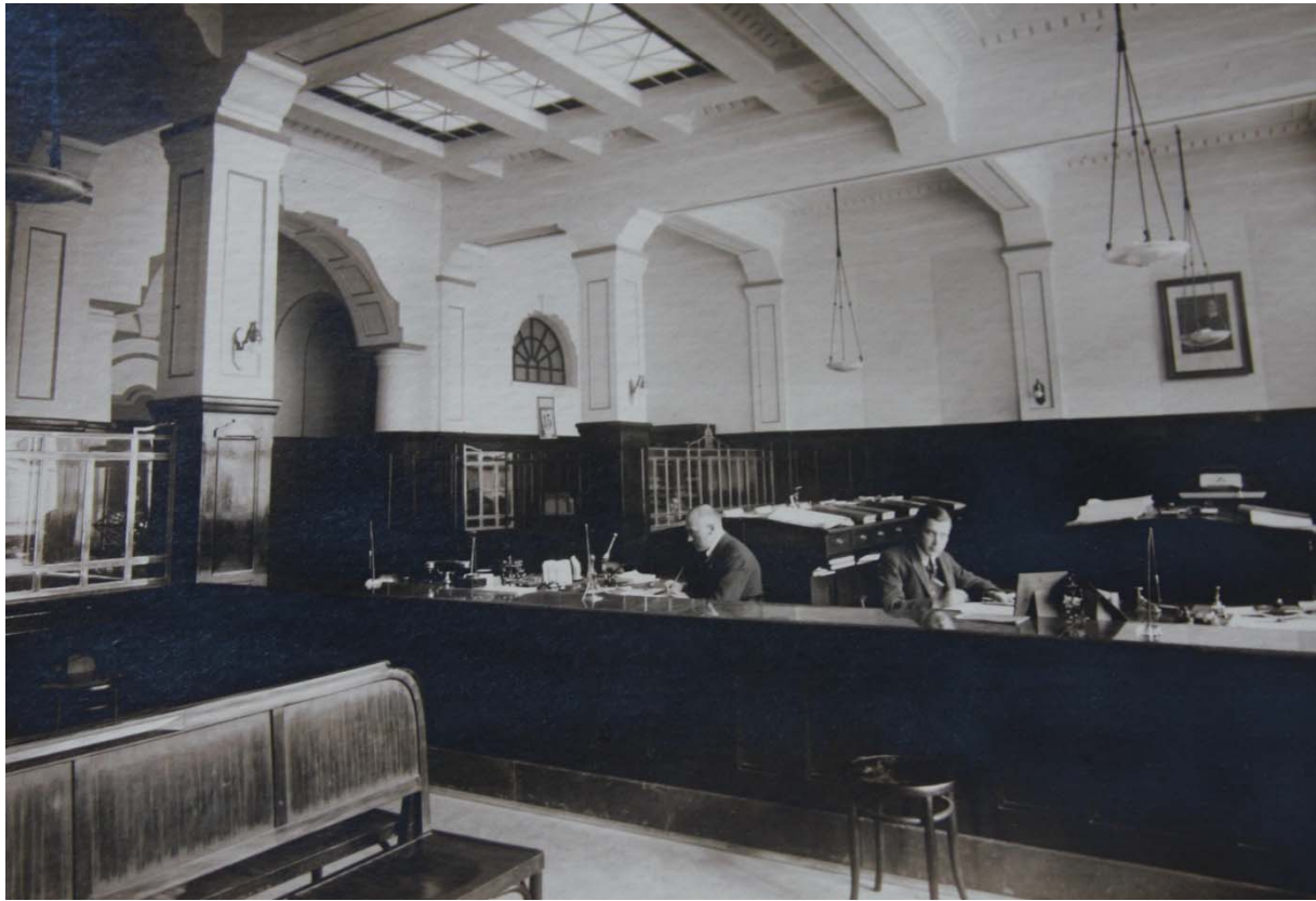
Figure 4. The branch of Tatra banka in Liptovský Mikuláš – the interior of the bank hall Source of the figure: [9]
