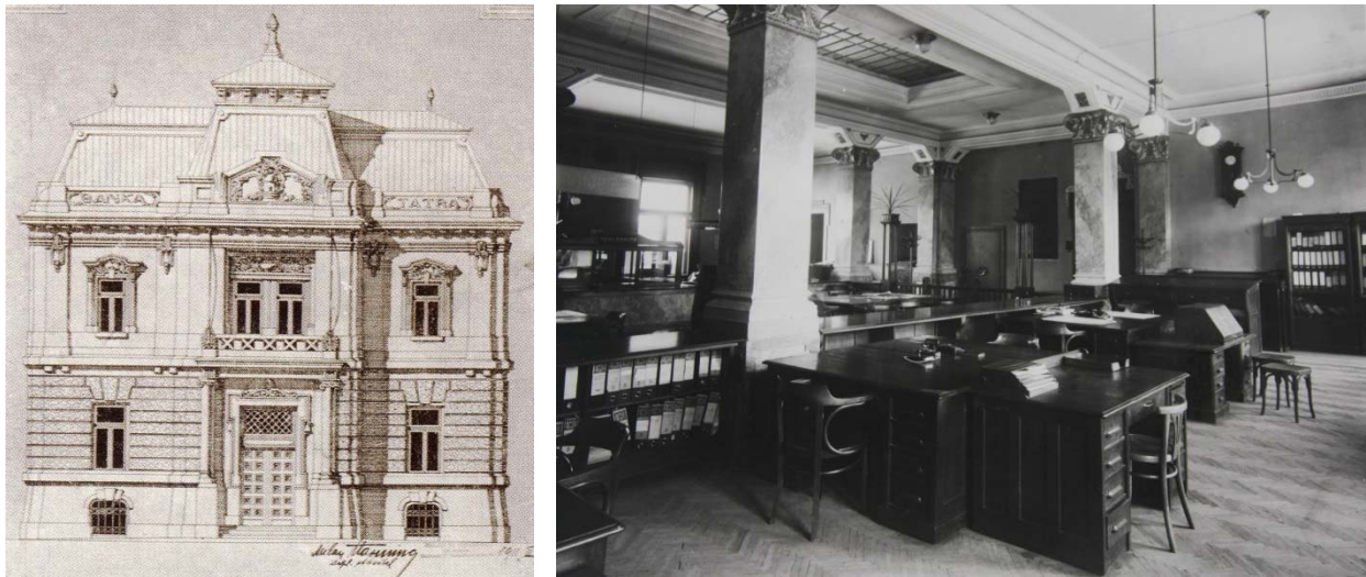
Figure 1. The Tatra banka in Martin – the entrance façade and bank hall, sources of the figures: [8], [9]
