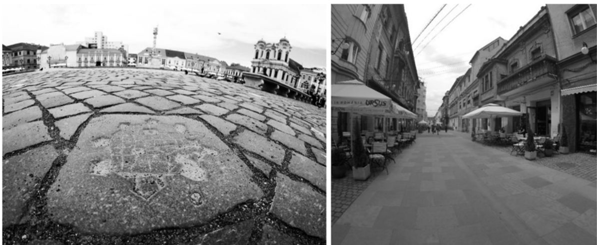
Figure 8. Union square and street from the district "Cetate" Timisoara, after the rehabilitation project
