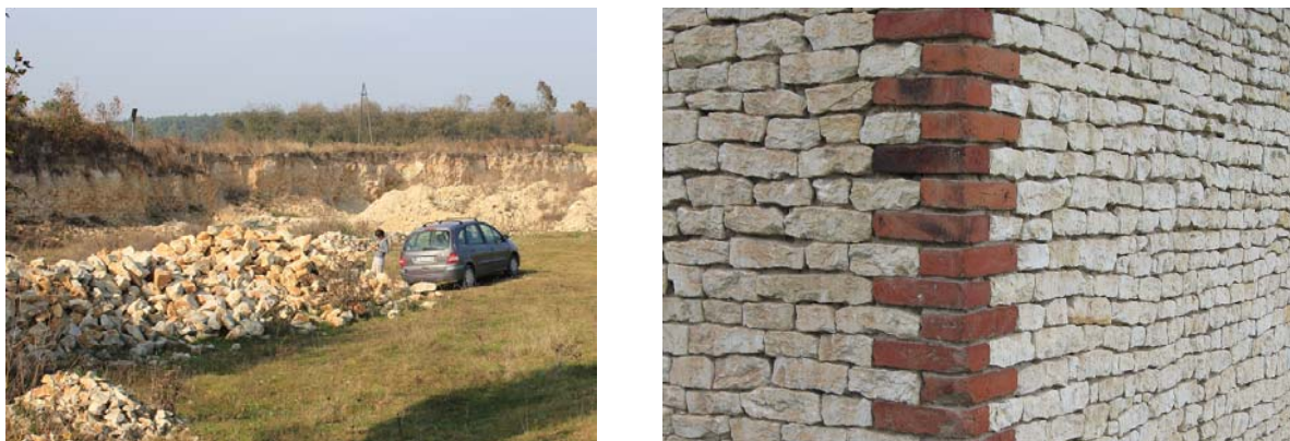
Figure 2. Quarry in Rożniatów (present condition) and typical method of using limestone in traditional rural architecture.
