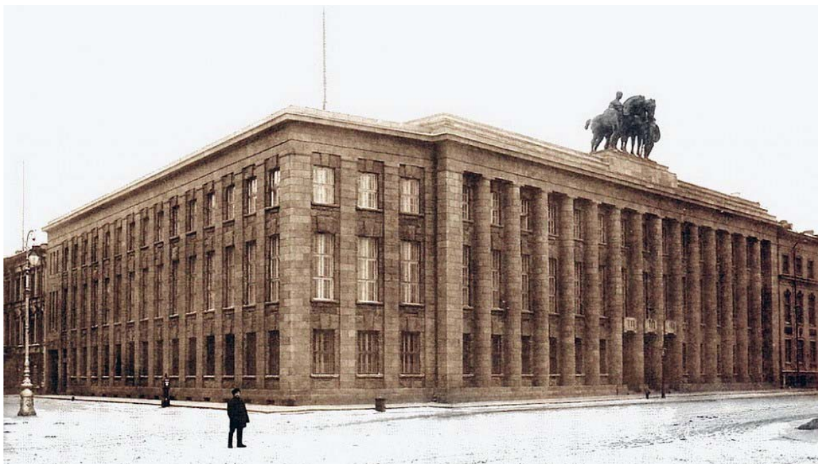
Figure 5. P. Behrens. The building of the German Embassy in St. Petersburg (1911-1913)
