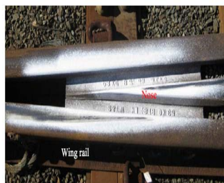
Figure 1. A standard turnout crossing nose [6]
