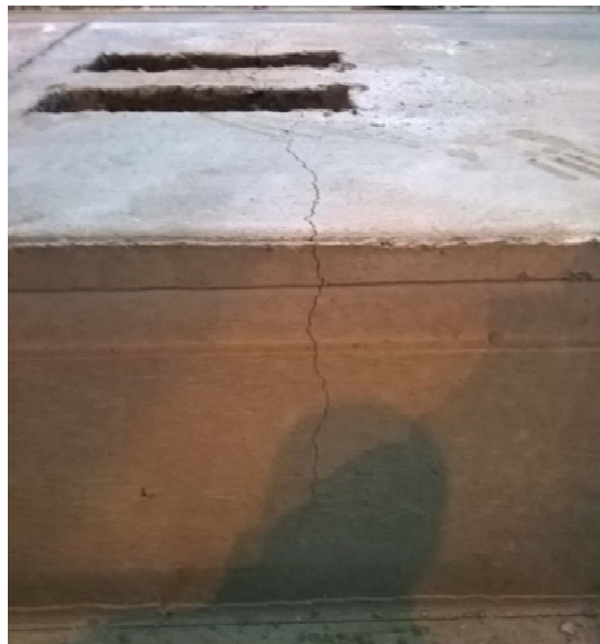
Figure 7. Cracks caused by shrinkage
