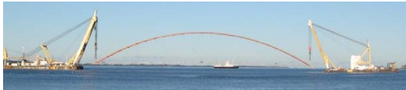
Figure 16. The 220m span of the Brandanger Bridge, moved to the pillars by big floating cranes.
