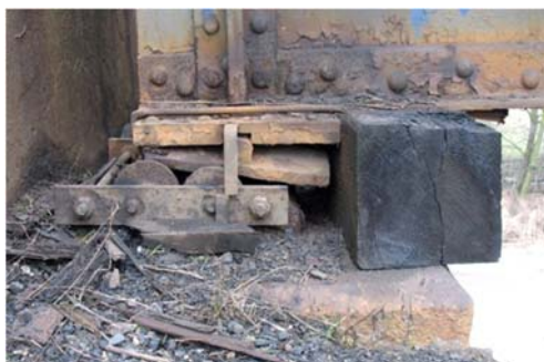
Figure 13. Additional temporary support of bridge span
