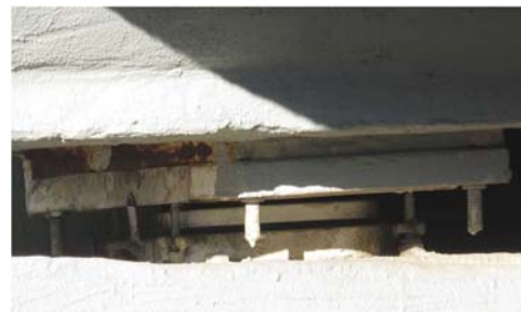
Figure 9. New Multi-directional pot bearing
