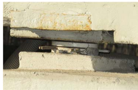
Figure 3. Pot bearing which replaced tangent bearing
