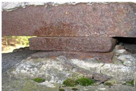
Figure 2. Corrosion of tangent bearing, cracks in ground beam
