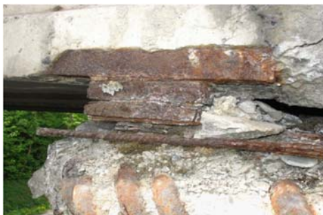
Figure 4. Corrosion and incorrect support of tangent bearing
