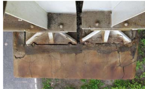
Figure 10. Permanent bearing, cracks in head of pillar (bearing bench)
