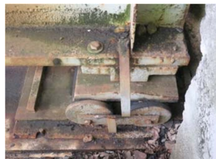
Figure 14. Niche in back wall and intentional displacement bottom plate of bearing
