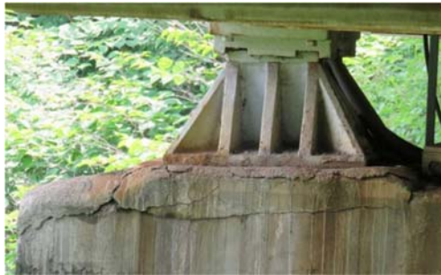
Figure 10. Permanent bearing, cracks in head of pillar (bearing bench)
