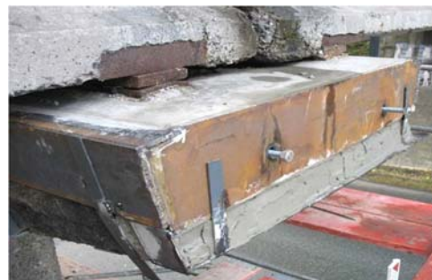
Figure 5. Repair of bridge bench and ground beams
