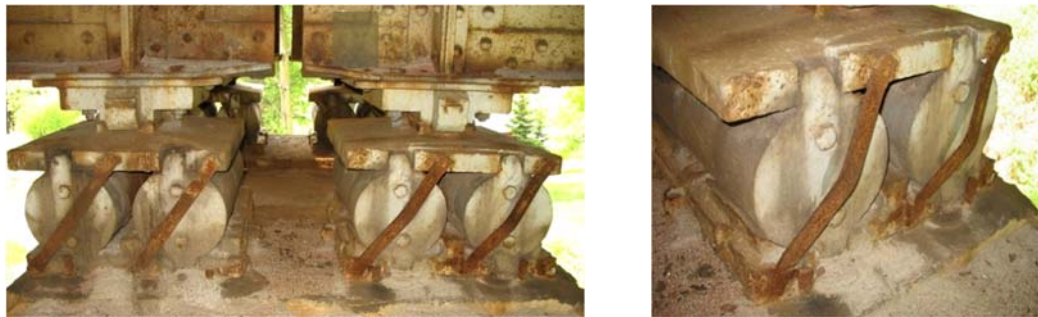
Figure 15. Amendment to the bearing scheme: blockade of one-way-sliding bearings
