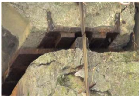
Figure 6. Old tangent linear bearing: freedom of displacements was restored by additional sheets
