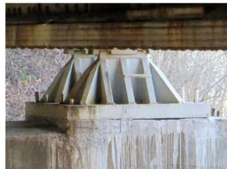
Figure 12. The permanent bearings on common steel plate
