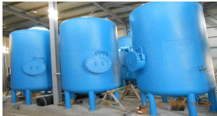
Figure 3. Sand filters + GAC filters
