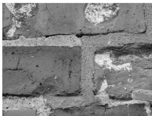
Figure 2. Subflorescence effect in a face brick in lens-shaped forms of sodium chloride
