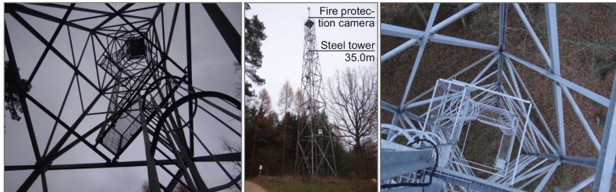
Figure 1. Overview and structural details of the lookout tower
