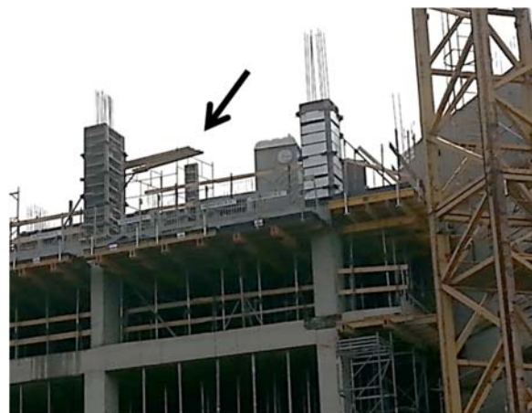
Figure 11. Incomplete Warsaw tower type scaffolding as a platform for concrete placers 15 metres above the ground, Poznań centre, 2018
