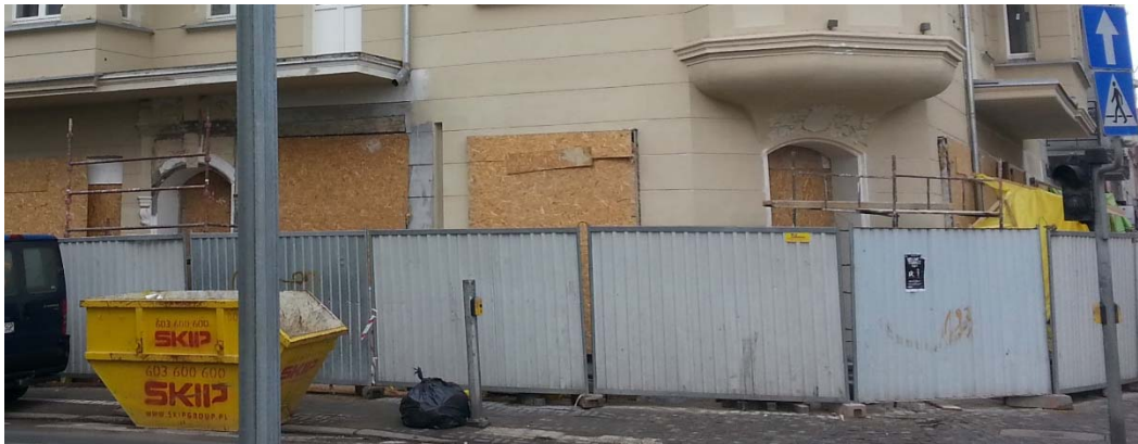
Figure 9. Makeshift platforms with missing elements covered with loose planks, main street in Poznań Old Town, 2018
