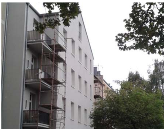
Figure 10. Small modular scaffolding – missing mid-rails and toeboards, Poznań centre, 2016
