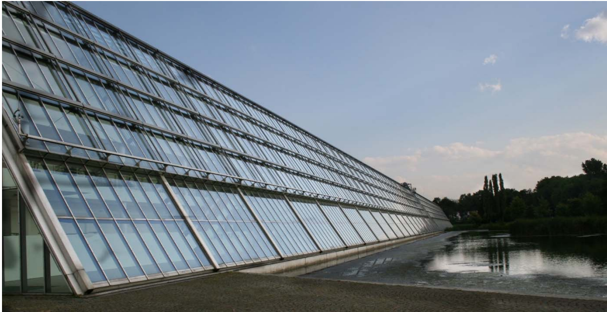
Figure 2. 300-metre-long glass passive façade of the technology center, covering a gallery that integrates individual wings of the building, is opened on greenery and an artificial lake
