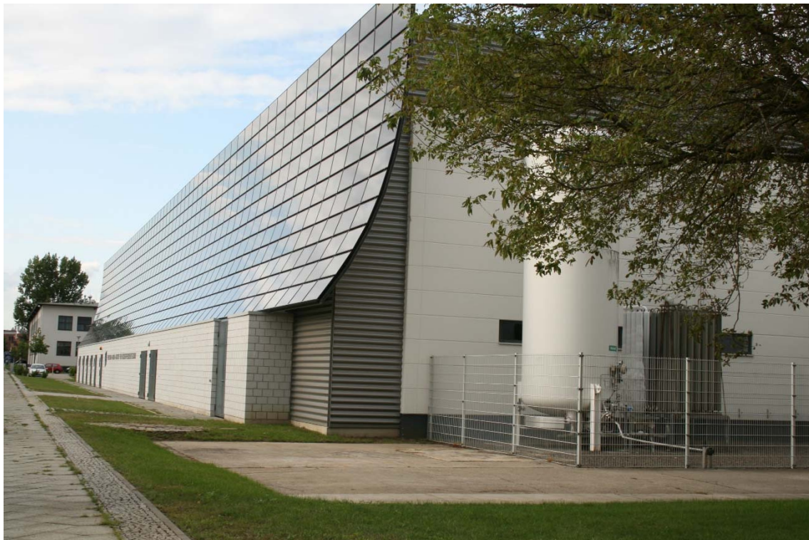
Figure 1. Dynamic façade. Building of the laboratory of Ferdinand-Braun-Institut, Leibniz-Institut High-Frequency Technology in WISTA Adlershof, Berlin, made of photovoltaic panels
