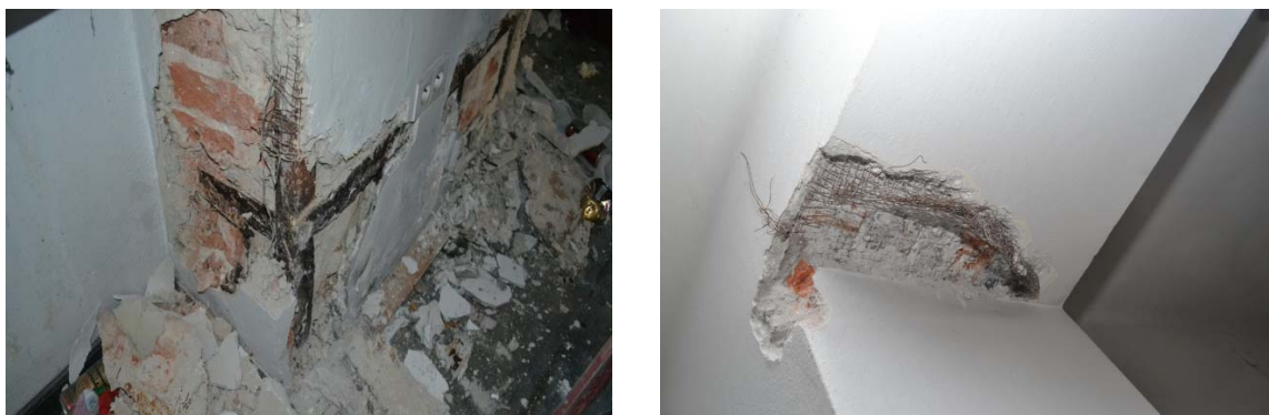
Figure 2. Structural reinforcements identified at the outcrops stage
