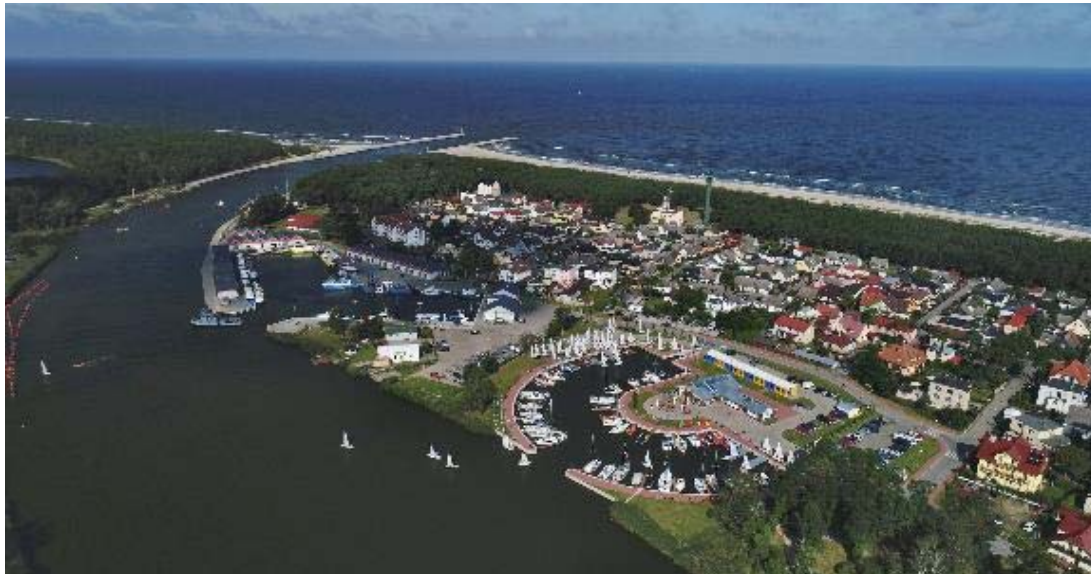
Figure 5. A new yacht port in Dziwnów opened in 2013 (compare with the figure 2). Source: MOSiK in Dziwnów.
