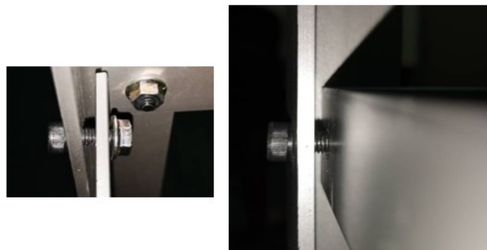
Figure 5. Detail image of damage condition on bolted joints.
