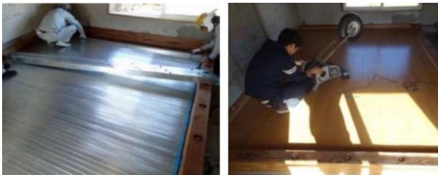
Fig. 6 Left: Placement of square bars in double floor; Right: Tire machine test.
