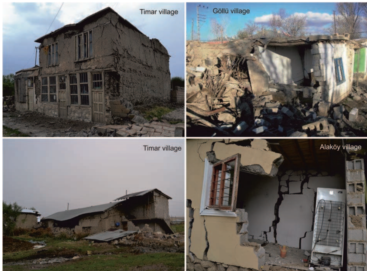
Figure 9. Damages to unreinforced masonry buildings on weak soils in the study area.
