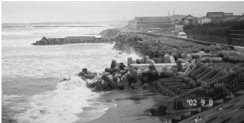
Figure 2. Photograph of Jinkoji coast taken at 17:00 on September 8, 2002 at tide level of 0.7 m above MSL before gravel nourishment.
