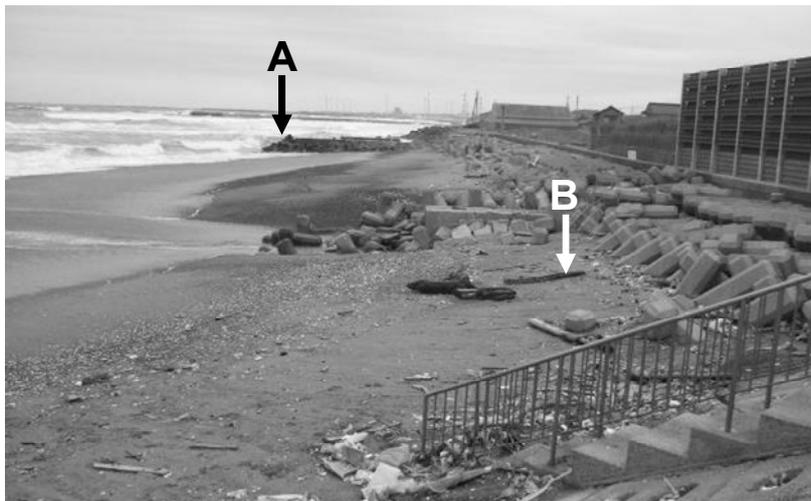
Figure 3. Photograph of Jinkoji coast taken at 16:00 on November 23, 2006 at tide level of 0.6 m above MSL after gravel nourishment.
