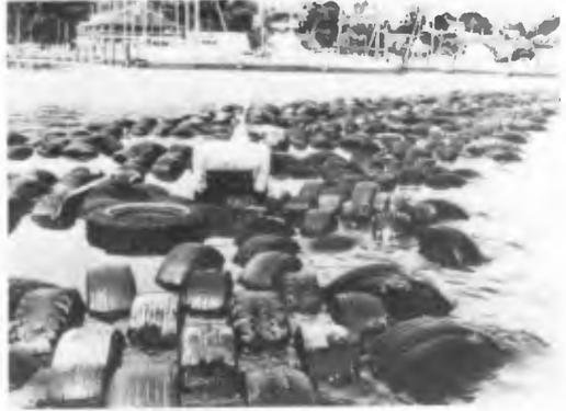
Figure 5. "Goodyear" type floating breakwater, Cranston, Rhode Island
