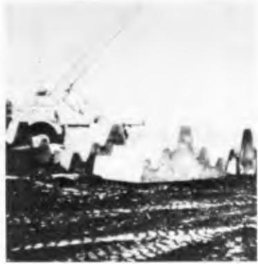
Figure 3. Campbell's precast breakwater units
