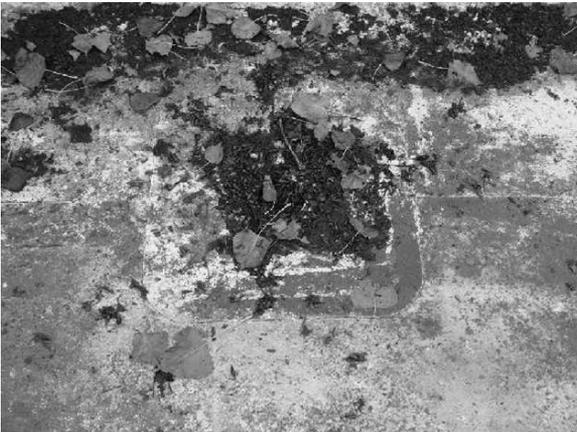
*Figure 2: Examples of blocked rainwater gullies*
