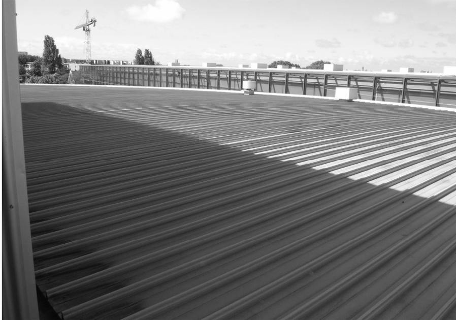
*Figure 6: An example of light-weight flat roof where already the detailing only (elevated trough roof sheeting under sufficient slope in combination with lower positioned roof gutters) prevents any form of rainwater ponding that could impair the structural safety and quality of the roof*
