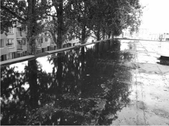
*Figure 2: Rainwater ponding, no emergency overflow in the roof up stands*
