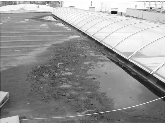
*Figure 4: Light street blocking the roof slope results in ponding*
