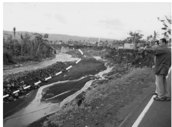
Fig. 9. Scoured river bank in Barangay Travesia, Guinobatan Town. The dotted line on the photo indicates the former location of the river bank. The collapsed rail track can be seen at the background
