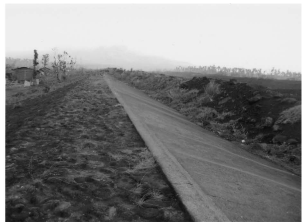
Fig. 8. Large channel created by the flowing lahar in Masarawag River is shown on the left photo. Photo on the right shows the river dike which successfully prevented the lahar from damaging residential houses on the west side of the dike
