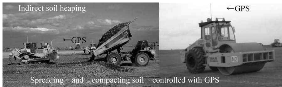
Fig. 20. Indirect soil heaping
