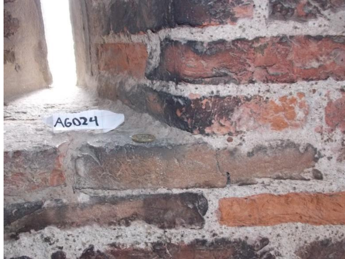
Figure 12. Above the brick marked with a coin, bricks cut to fit into a window overlook are pictured.
