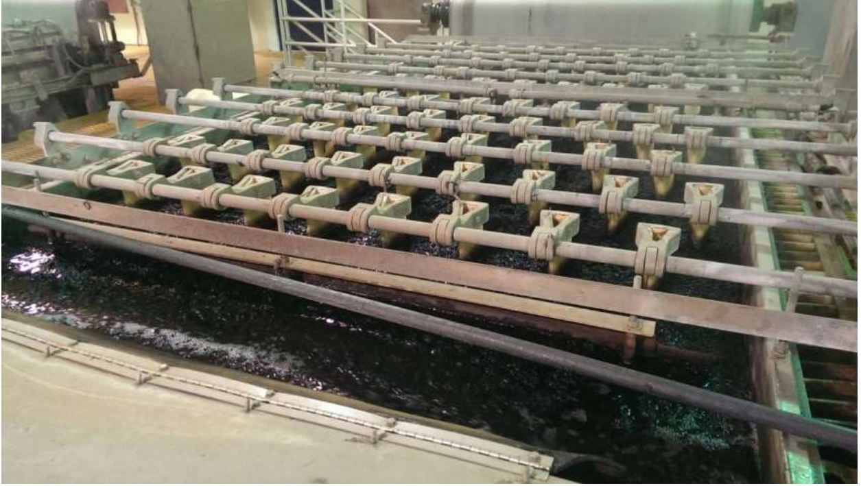
Figure 1. Plows in the gravity drainage zone on a belt filter press processing anaerobically digested sludge – Photo taken with permission at the Fresno/Clovis Regional Wastewater Treatment Facility in Fresno, CA
