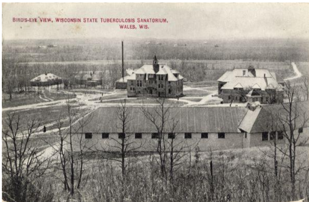
Fig 2. Elevated View of the Wisconsin State Sanatorium. 21
