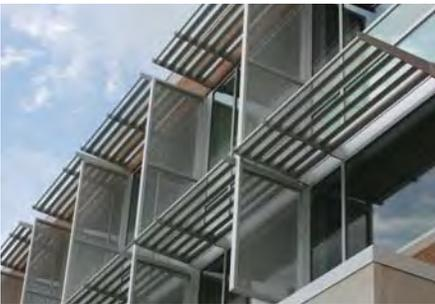
ROOFS AND SHADING DEVICES SHOULD BE PROVIDED ON SOUTHERN FACADES
