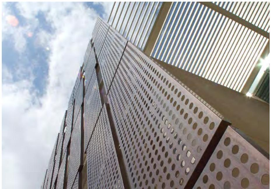
FACADES SHOULD ADMIT DAYLIGHT AND PREVENT EXCESSIVE HEAT GAIN
