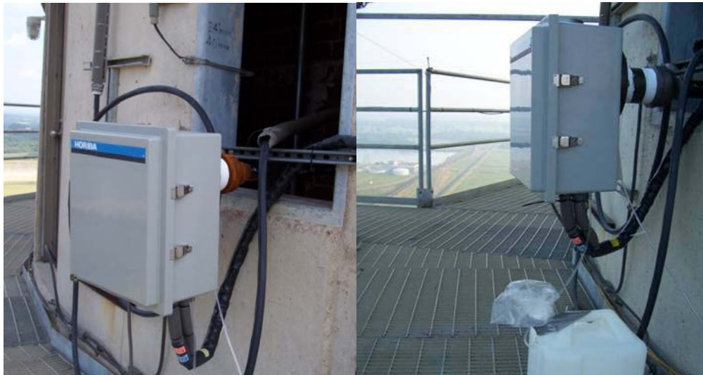
Figure 2.3.3.2 Hg-CEM system installation at stack test platform
