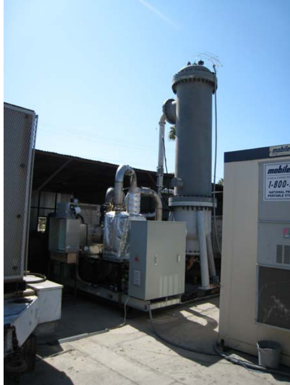
Figure 6 Thermal Oxidizer Attached to Elliot Microturbine
