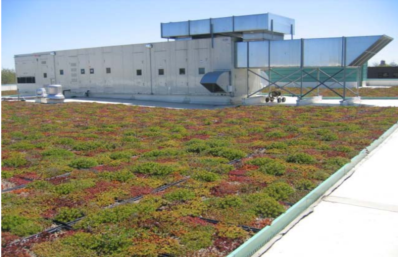
Figure 6 The high efficiency roof top unit and green vegetated roof
