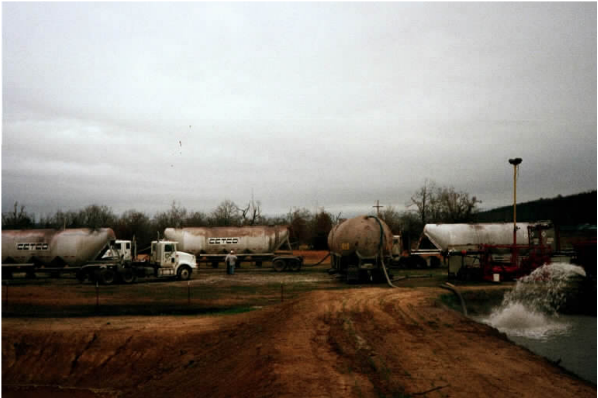
AIT staging area. CCB transport trucks download fluidized bed combustion ash for the injection slurry.
