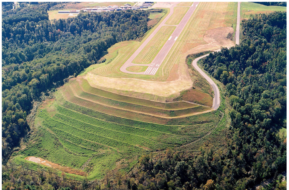
FGD byproducts from a nearby power plant were used to expand this runway at Pennsylvania's Rostraver Airport.
