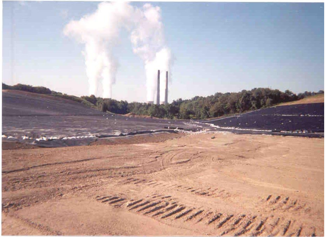
A CCP landfill under construction in the northeastern U.S.
