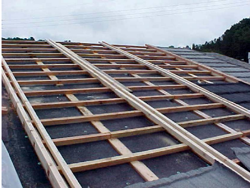
Fig. 4. Construction of the roof deck showing battens and counter-battens for attaching the slate tile and the parapets used to prevent cross flow from one test roof to another.
