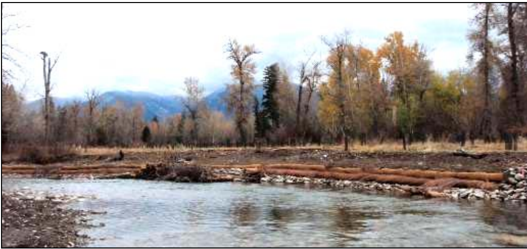
Figure 8. Photograph showing a typical vegetated soil lift sequence on an outer meander bend. Vegetated soil lifts were installed in conjunction with other bank protection treatments such as engineered log jams.
