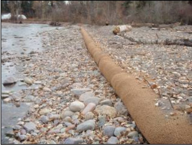
Figure 9. Completed wrapped coir log with vertically installed willow cuttings.
