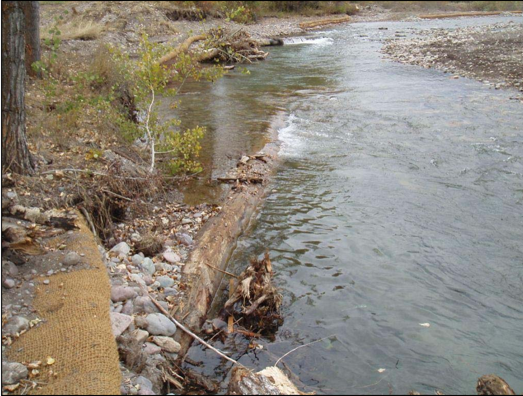
Figure 7. Log vane after channel construction.
