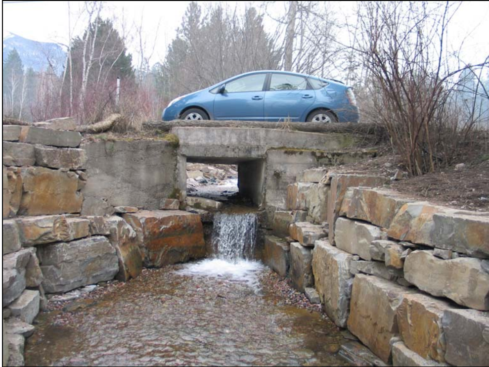
Figure 1. Constructed passage barrier near the mouth of Skidoo Creek, 2008.
