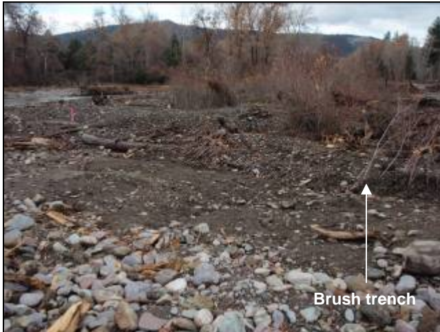
Figure 11. Brush trench incorporates woody debris, willow cuttings and mature plant material to create floodplain roughness and microsites for woody vegetation establishment.
