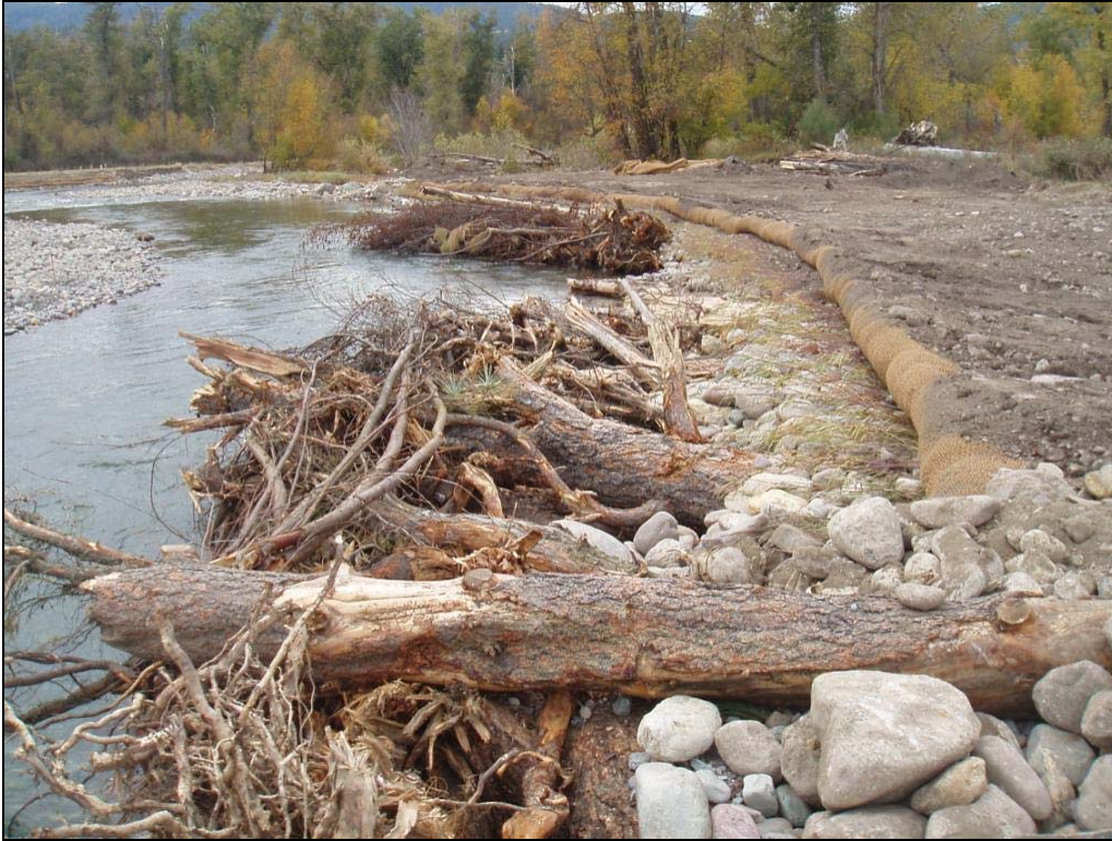
Figure 6. Engineered log jam tied in with streambank bioengineering.
