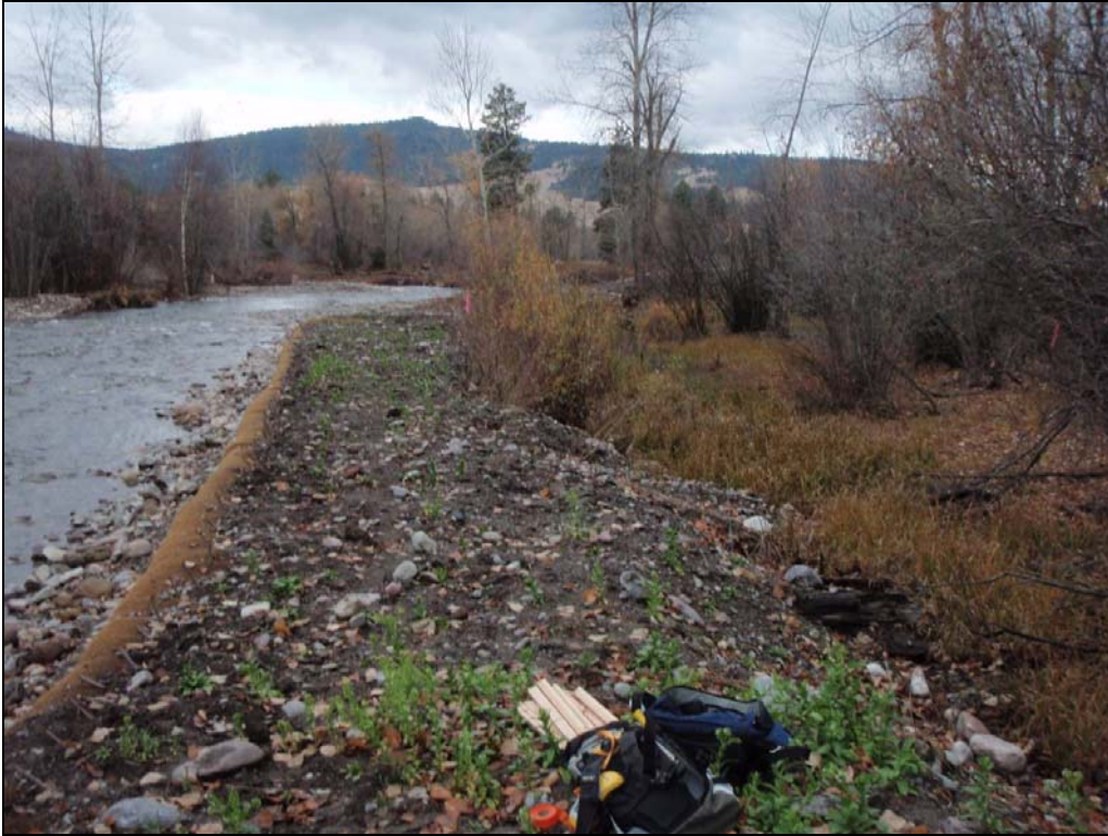
Figure 14. Stinger planted riparian tree and shrub seedlings behind a wrapped coir log.
