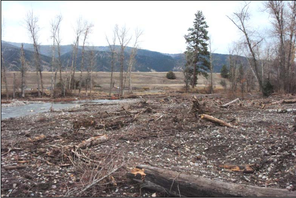
Figure 13. Floodplain microtopography including swales, woody debris and a rough, finished surface.
