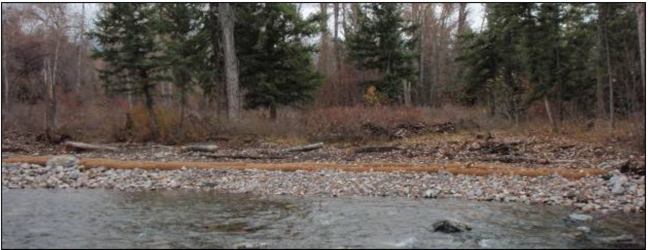
Figure 10. Photograph shows double layer anchored coir log tying into existing vegetation at the downstream end (at photo right).
