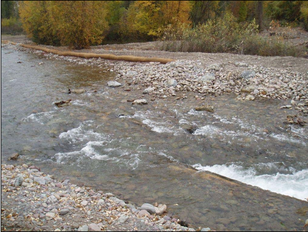
Figure 5. Submerged boulder energy dissipater during construction Bank Protection
