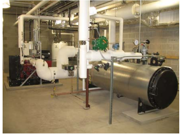
Figure 4. Heat recovery steam generator
