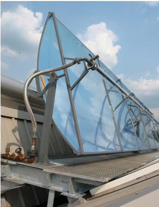
Figure 5. Parabolic trough solar thermal receiver
