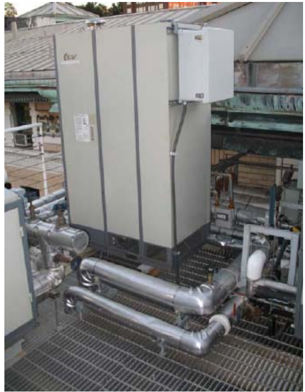
Figure 6. Two stage absorption chiller
