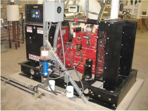
Figure 3. BioDiesel fueled engine generator
