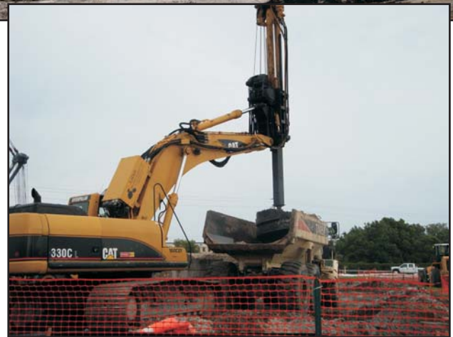
Placing soil from the large-diameter auger into a dump truck at the 4.5 Acre Site.
