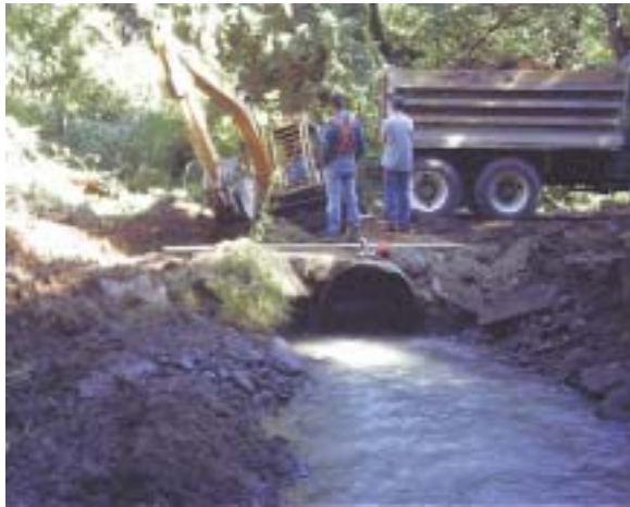
Figure 1. Excavation around the existing culvert was accomplished without disturbing the culvert or the stream. There was an average of 5' of fill on top of the culvert. This photo shows the culvert after most of the fill has been removed above the culvert.
