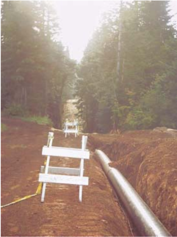
Figure 1. A section of the Hutson Extension, comprised of 48" HDPE pipe. This shows the crossing of West Fork Evans Creek. Note the native grasses spread to control erosion on the disturbed areas. This is before the system was hooked up and pressurized.
