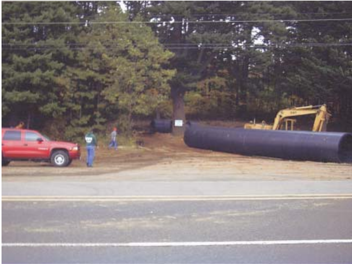
Figure 2. An example of a section of 72" HDPE pipe before being installed in the canal alignment.
