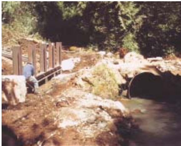
Figure 2. Bridge supports were installed and welded without disturbing the culvert and stream.
