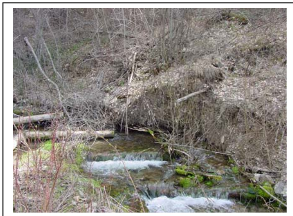
Some Iron Creek log structures washed out during high water event of 1996-97 causing bank to undercut. Will continue to monitor may need to be repaired.
