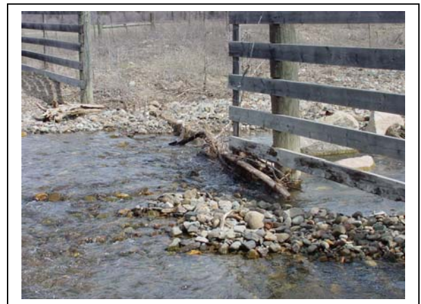
Gates on South Nanamkin Creek collected debris and altered channel during high water event of 1996-97. Gates removed will not be used again.
