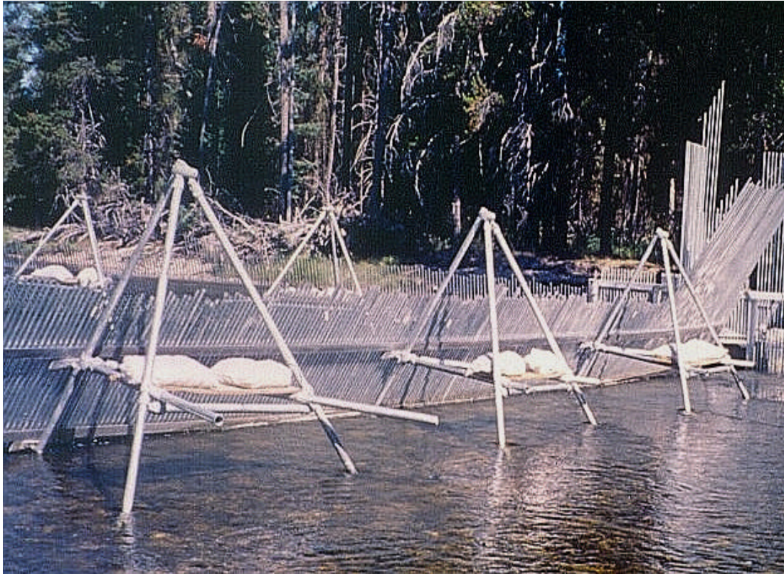
Figure 4. Temporary tripods, pickets and stringers used on the fish guiding fence.
