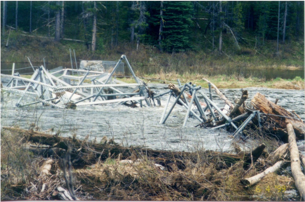
Figure 25. Failed Secesh River fish counting station.
