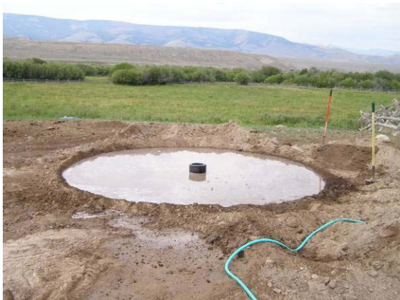
Trough #4 location before concrete is poured.
