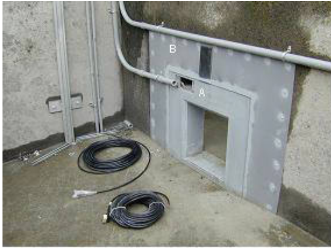
Appendix Figure A1. Photo taken during the installation of PIT-tag detection equipment into the Washington Shore Fish Ladder at Bonneville Dam. The antenna housing is labeled with the letter A at the approximate location of the connector inside the recessed access chamber. The aluminum shield is labeled with the letter B.
