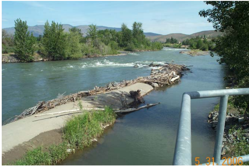
Figure 8. View Upstream from Glead of Concrete Arm and Remnants of 2005 Push-Up Dam that Form the Glead Diversion, May 2006
