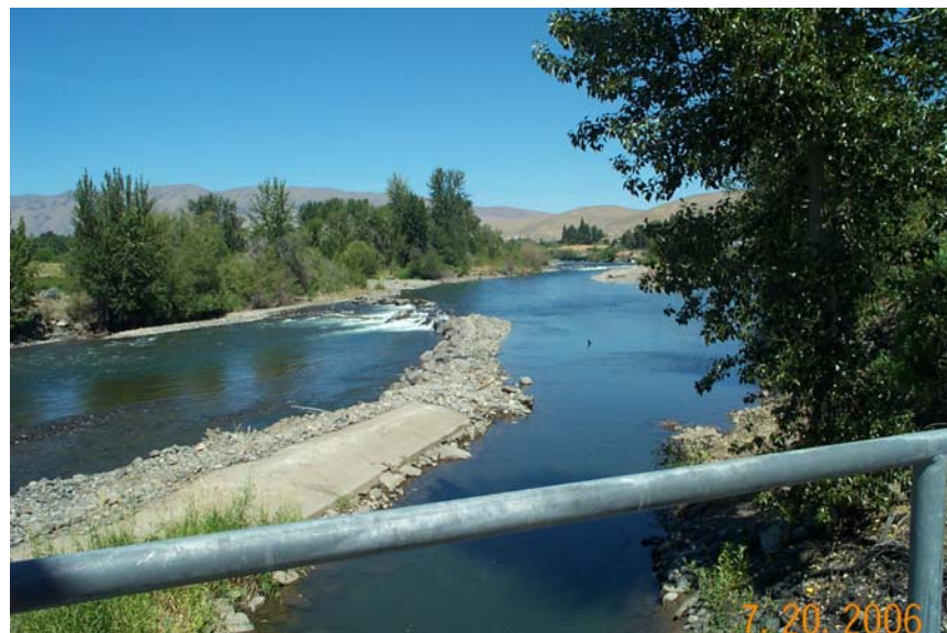
Figure 9. View Upstream from Glead of Concrete Arm and New Push-Up Dam that Form the Glead Diversion, July 2006
