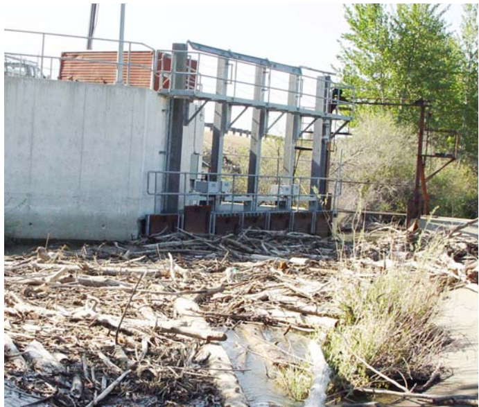
Figure 1. View Downstream at Log Jam and Protective Metal Plates on May 1, 2006. Control gate is not raised.
