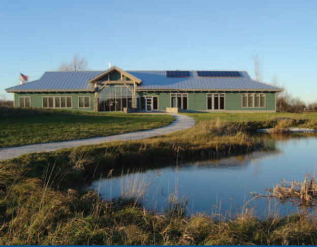
The Missisquoi National Wildlife Refuge Headquarters and Visitor Contact Station showcases renewable energy with a geothermal HVAC system, 15 kW PV array, 10 kW wind turbine, and clean-burning wood stove.
