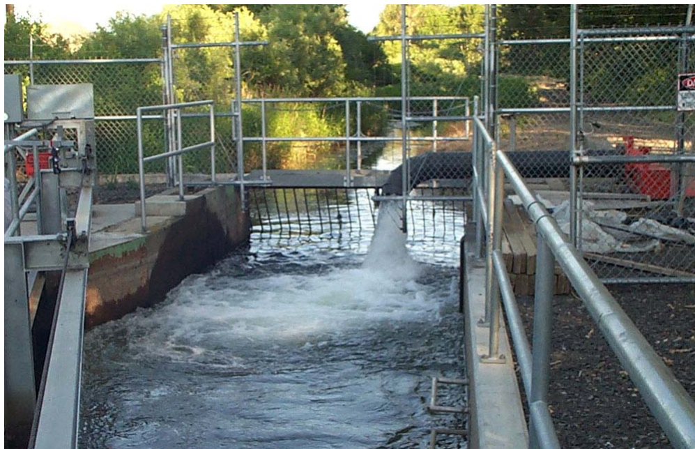
Figure 58. Water being piped in from the Old Union screen site into the Fruitvale forebay. View upstream from bypass.
