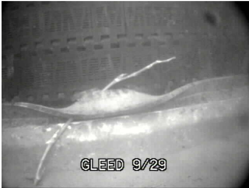
Figure 81. Stick twisted through a bottom seal at Gleed
