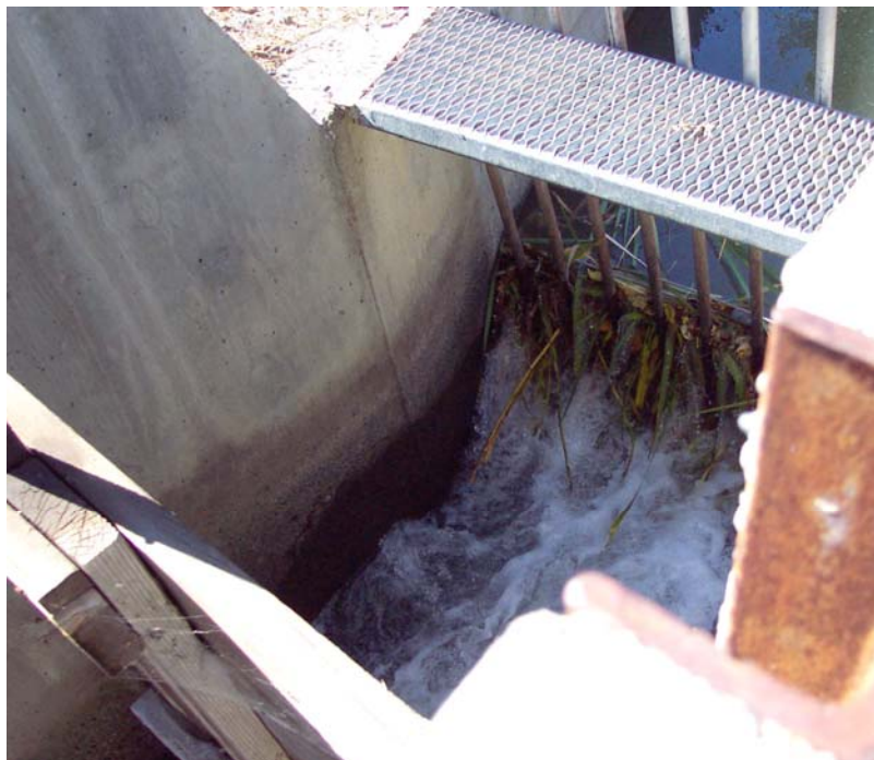
Figure 37. Upper trash rack at Powell-LaFortune partly blocked with debris. Approximately 12 in. of head loss are visible.
