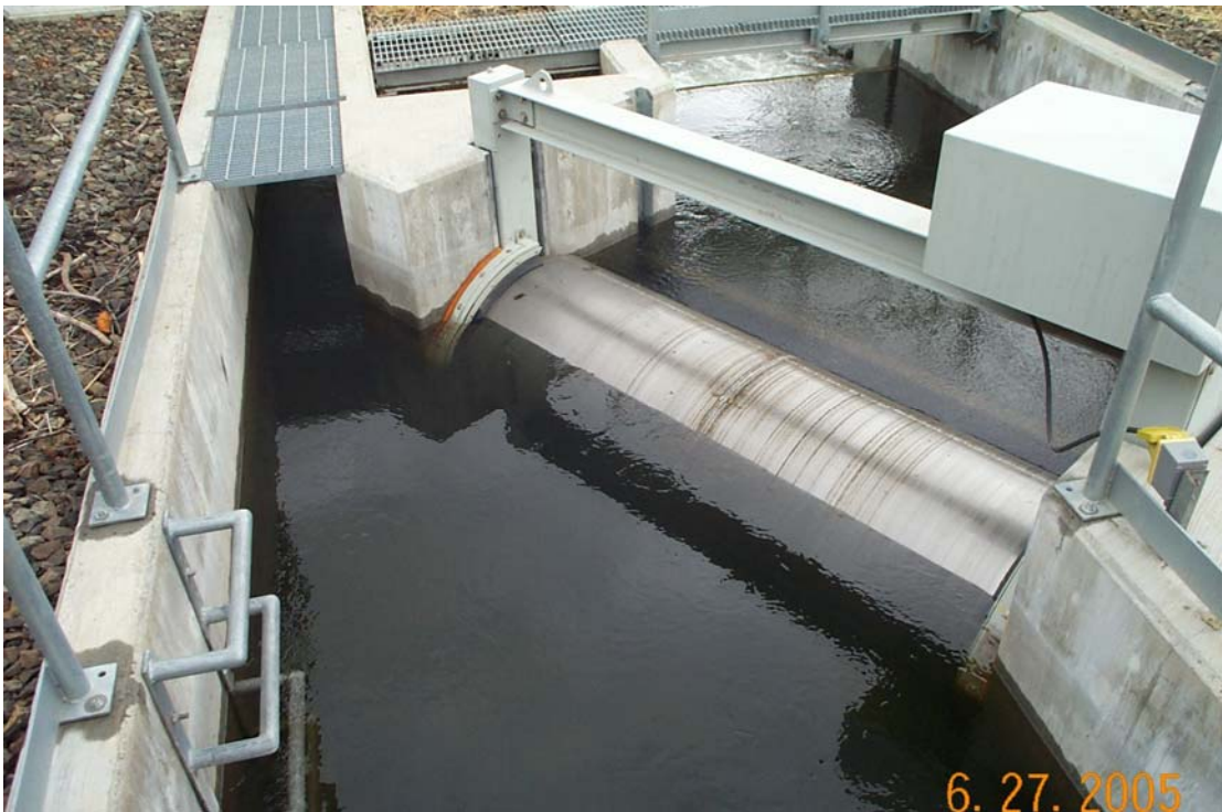
Figure 15. Drum and bypass entrance at Huntsville Mill site
