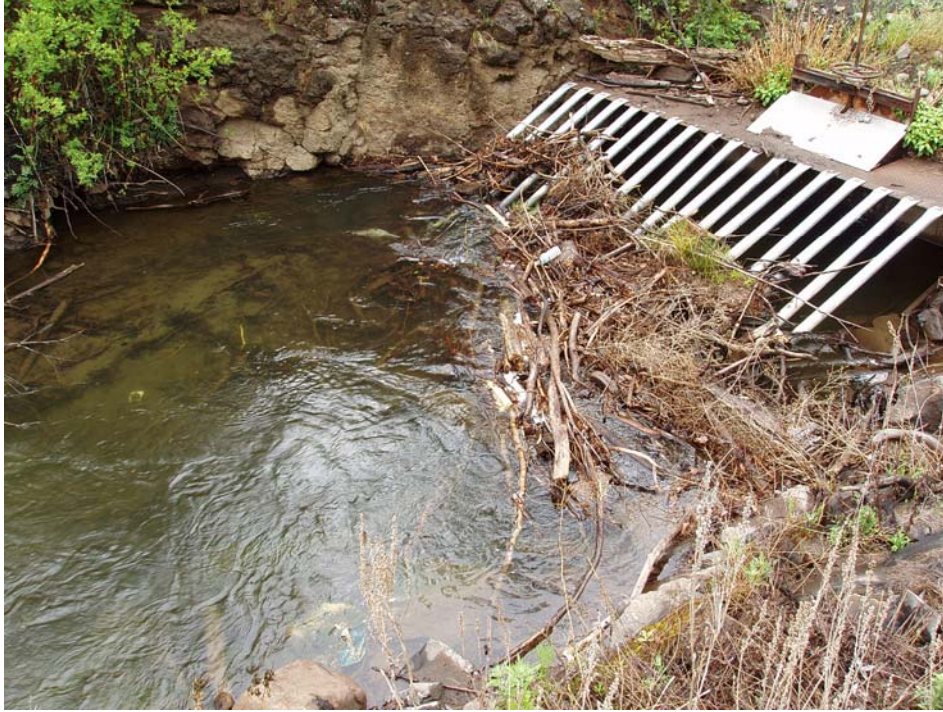
Figure 21. John Cox trash rack, laden with debris
