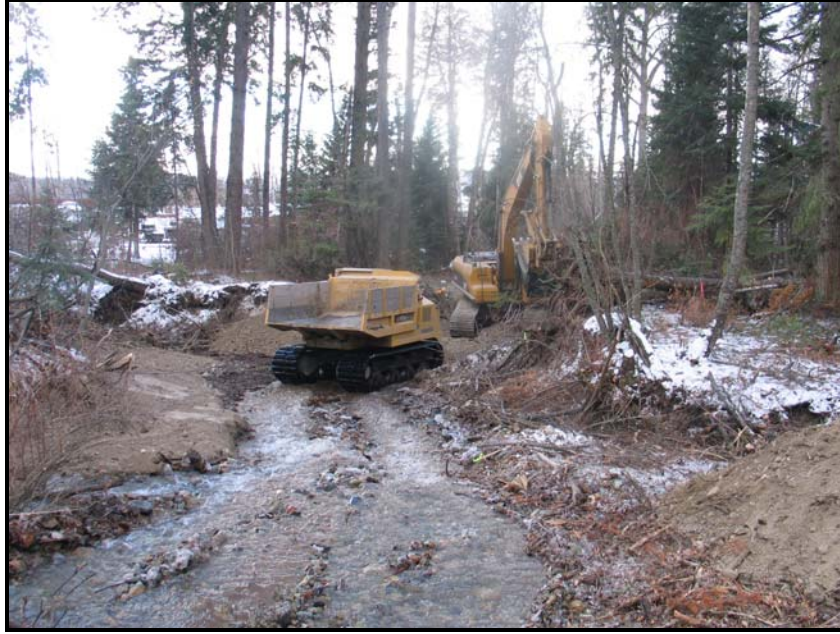
Figure 14. Hell Roaring Creek during channel reconstruction, December 2007.
