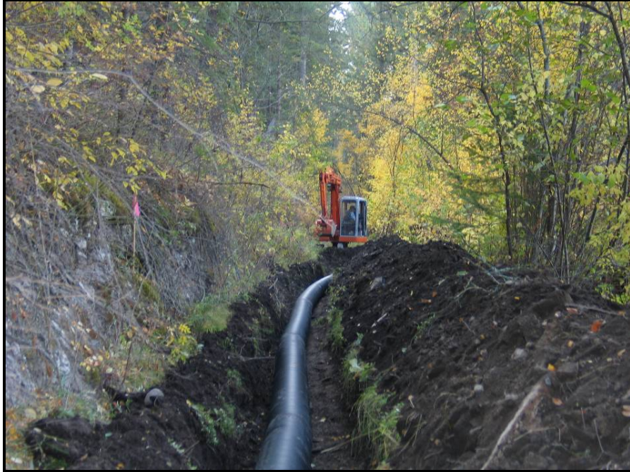
Figure 19: Pipe installation within irrigation ditch from Valley Creek, 2007.
