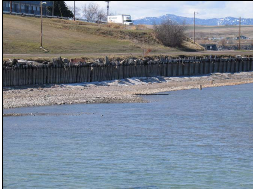
Figure 7. Failing wooden seawall at Salish Point on Flathead Lake.
